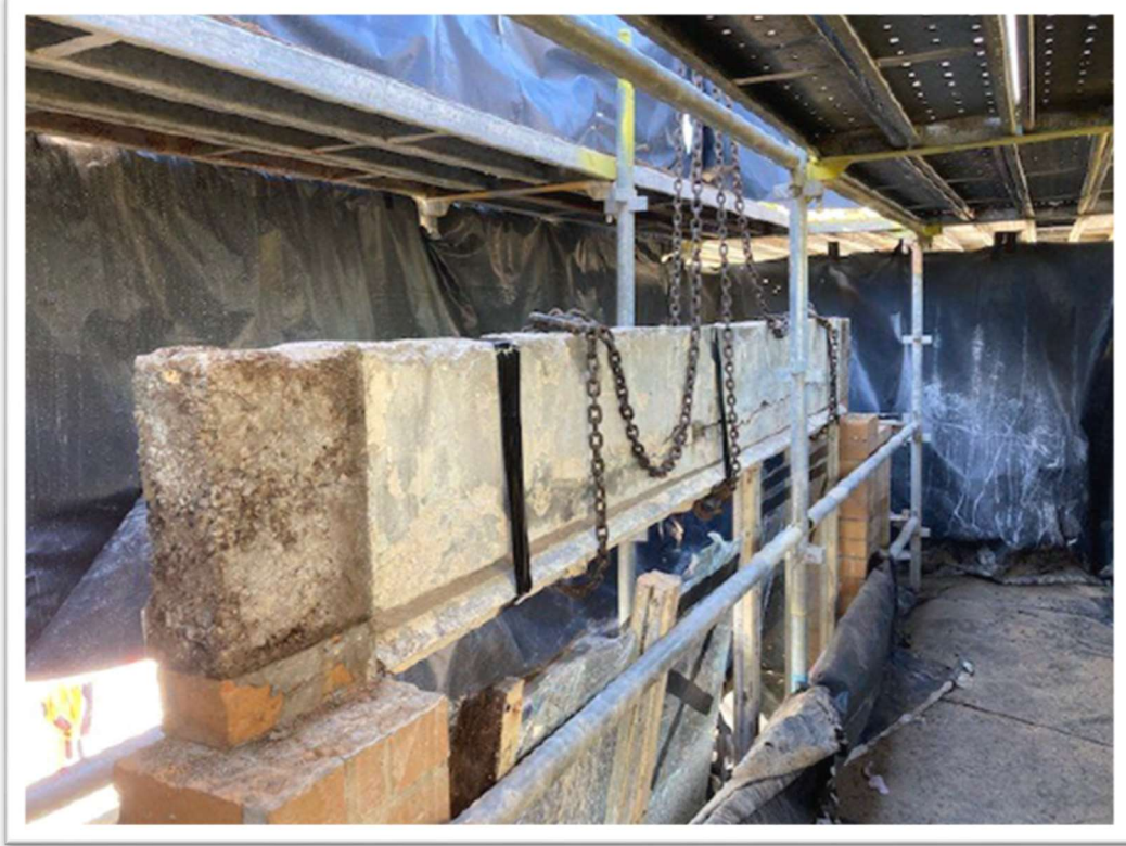
Figure 9. CEMENT BASED MORTAR (SILICA) BEING CAREFULLY REMOVED USING A WET SAW TO PRESERVE THE HERITAGE BRICKS FOR RECONSTRUCTION OF PORTICO.
