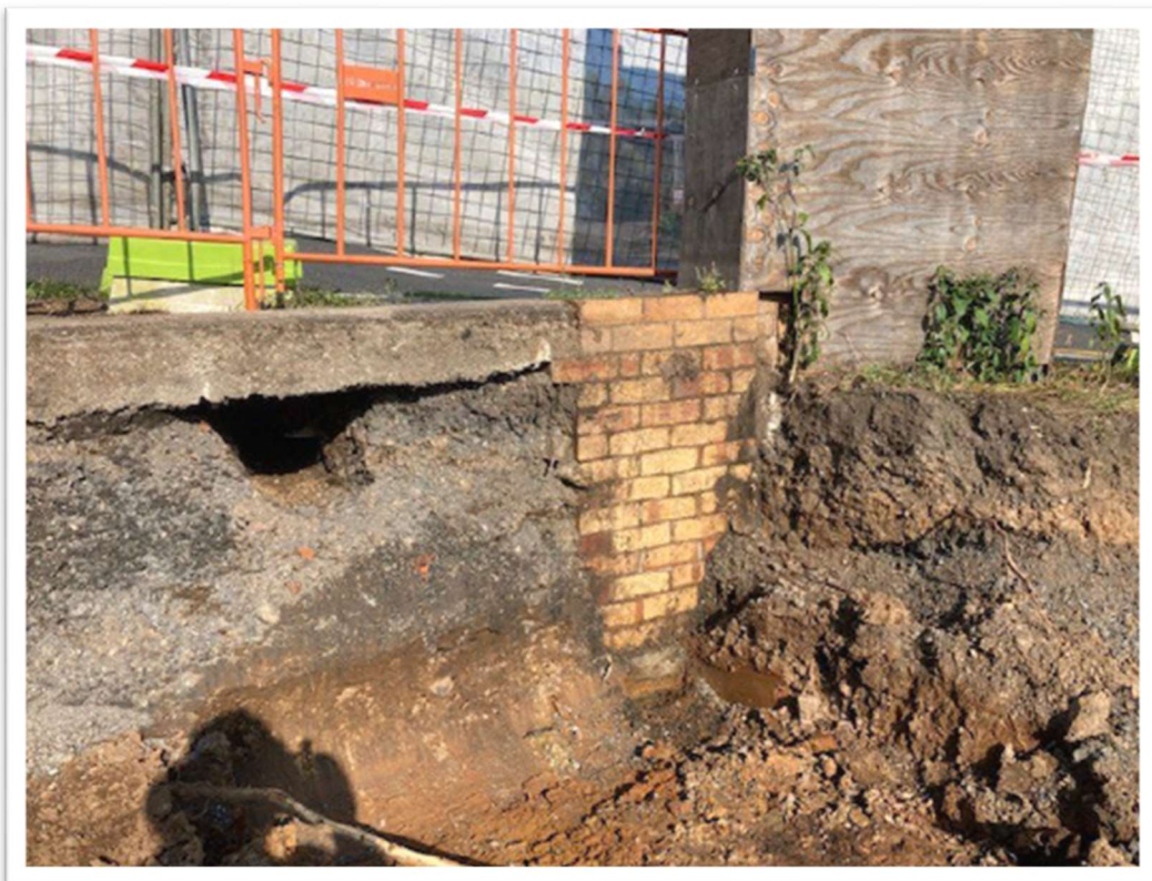
Figure 26. PLYWOOD HOARDING AND SUB SURFACE BRICK AND CONCRETE FOUNDATIONS OF GATES PRESERVED
