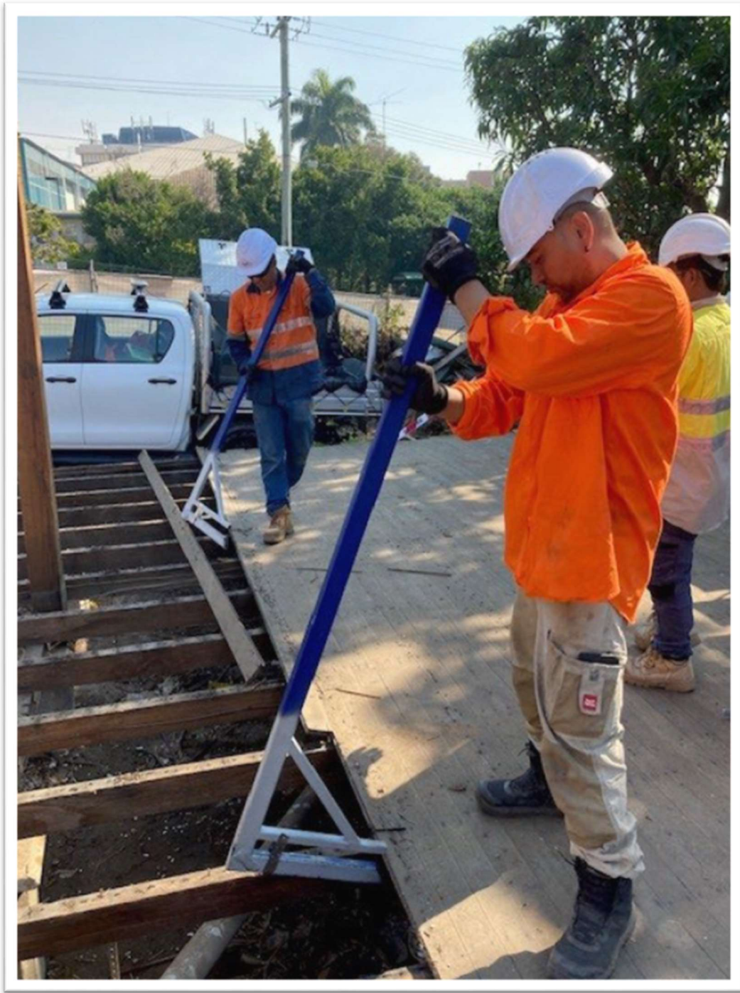
Figure 30. NON-DESTRUCTIVE METHOD OF FLOORBOARD RECOVERY
