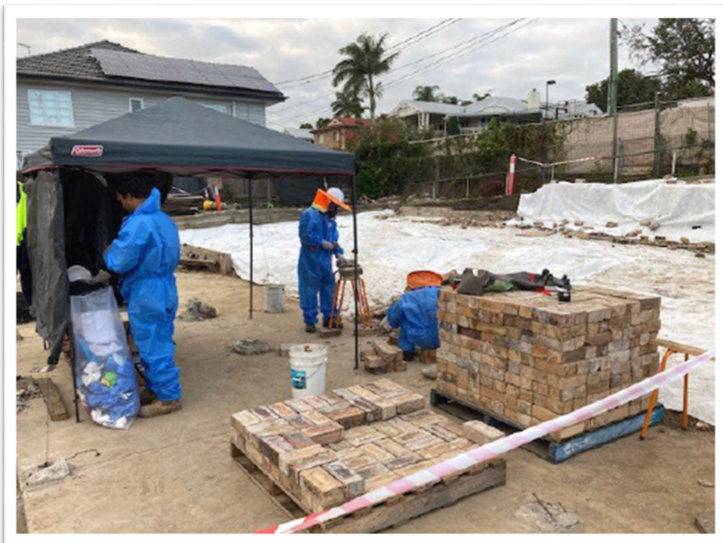
Figure 15. MANUAL CLEANING / RECOVERY PROCESS OF THE HERITAGE LIST BRICKS THAT WILL BE RE-USED IN INTERPRETIVE HERITAGE STRUCTURE IN PARK
