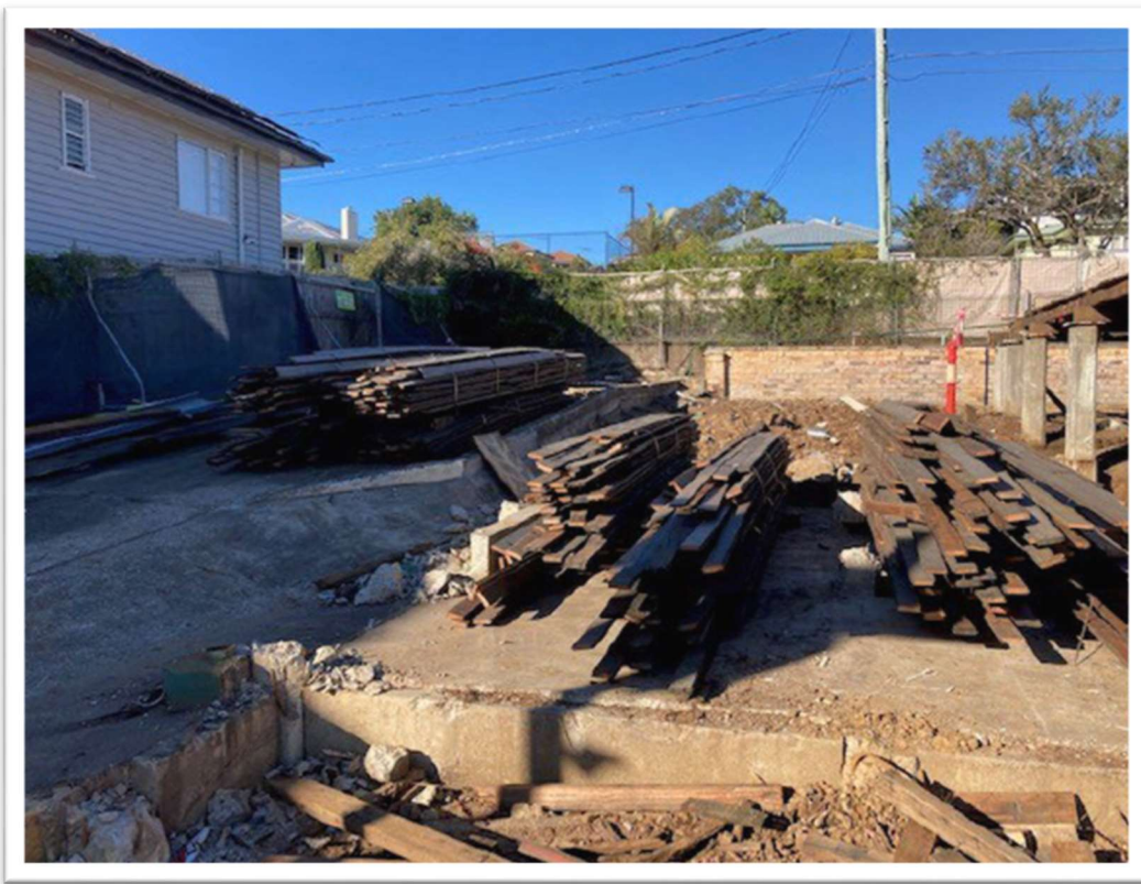
Figure 32. SALVAGED FLOORING TIMBER FOR RE-USE IN LEGACY HOUSE, READY TO BE DE-NAILED
