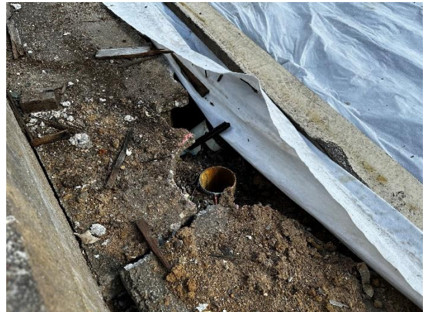
Photo 4: Central drain surround following removal works.
