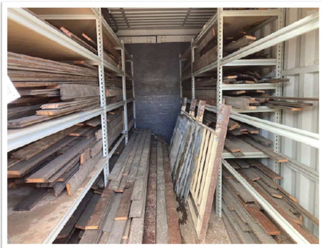
Figure 19. SHIPPING CONTAINER WITH PORTICO BALUSTRADE IRONWORK STORED ALONG WITH 500M2 OF SALVAGED HARDWOOD FLOOR BOARDS, DE-NAILED AND DESTINED FOR RE-USE IN THE NEW LEGACY HOUSE.
