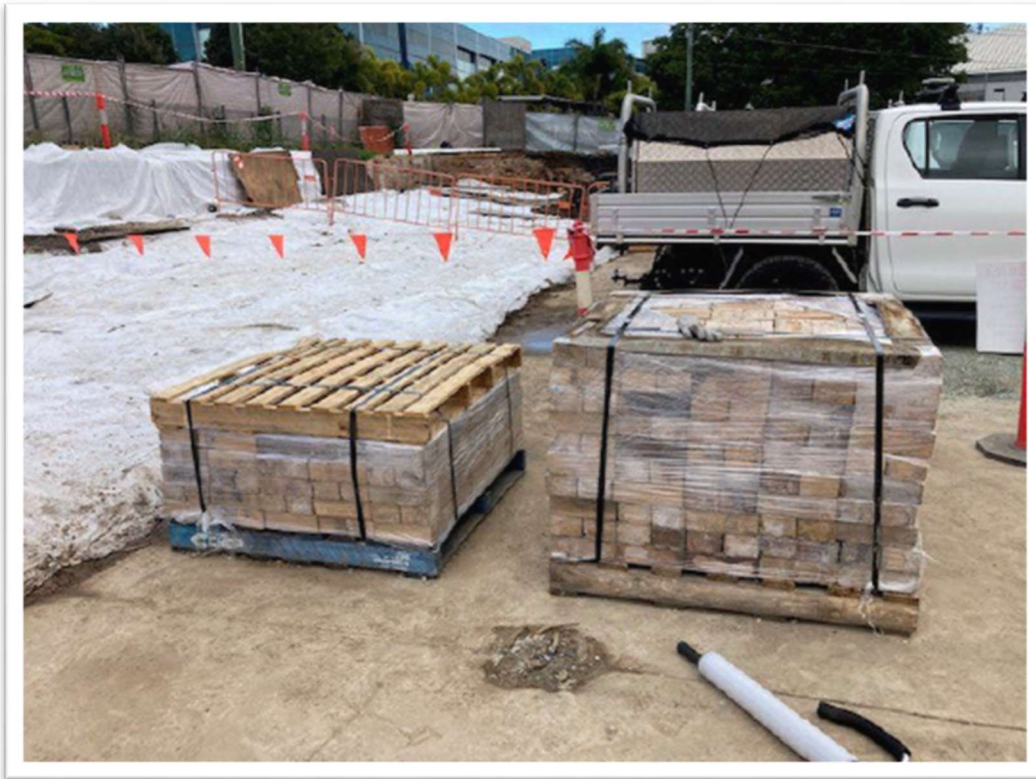
Figure 18. RECOVERED PORTICO BRICKWORK, CLEANED OF MORTAR, AND PALLETISED READY FOR STORAGE.
