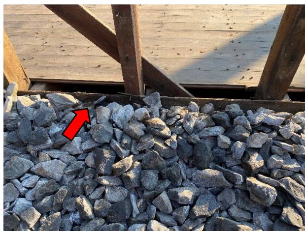
Photo 8: Residual Lead containing paint - Accommodation block, S lower wall – lower course of weatherboard panels below ground level.
