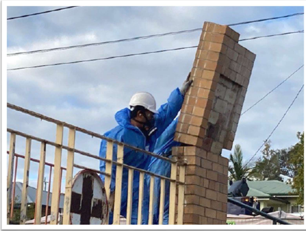
Figure 12. CONTROLLED SEPARATION OF THE BRICK COLUMNS. THESE SECTIONS WERE SEPARATED BY A HORIZONTAL “WET” SAW CUT UNDER SILICA CONTROLLED CONDITIONS AND MANUALLY DIRECTED ONTO SOFT SOILS FOR FURTHER BRICK SEPARATION AND SALVAGE.
