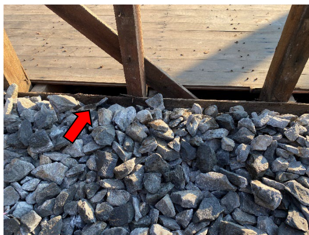
Photo 8: Residual ACM - Accommodation block, S lower wall – lower course of weatherboard panels below ground level.
