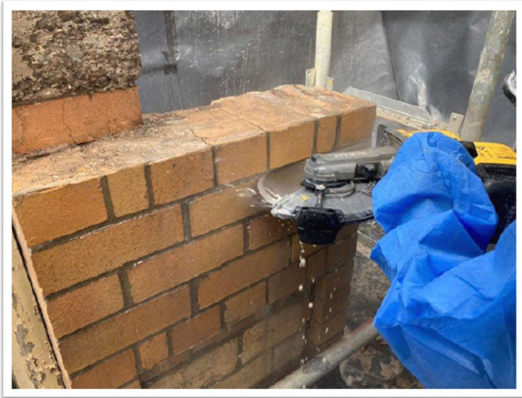
Figure 9. CEMENT BASED MORTAR (SILICA) BEING CAREFULLY REMOVED USING A WET SAW TO PRESERVE THE HERITAGE BRICKS FOR RECONSTRUCTION OF PORTICO.
