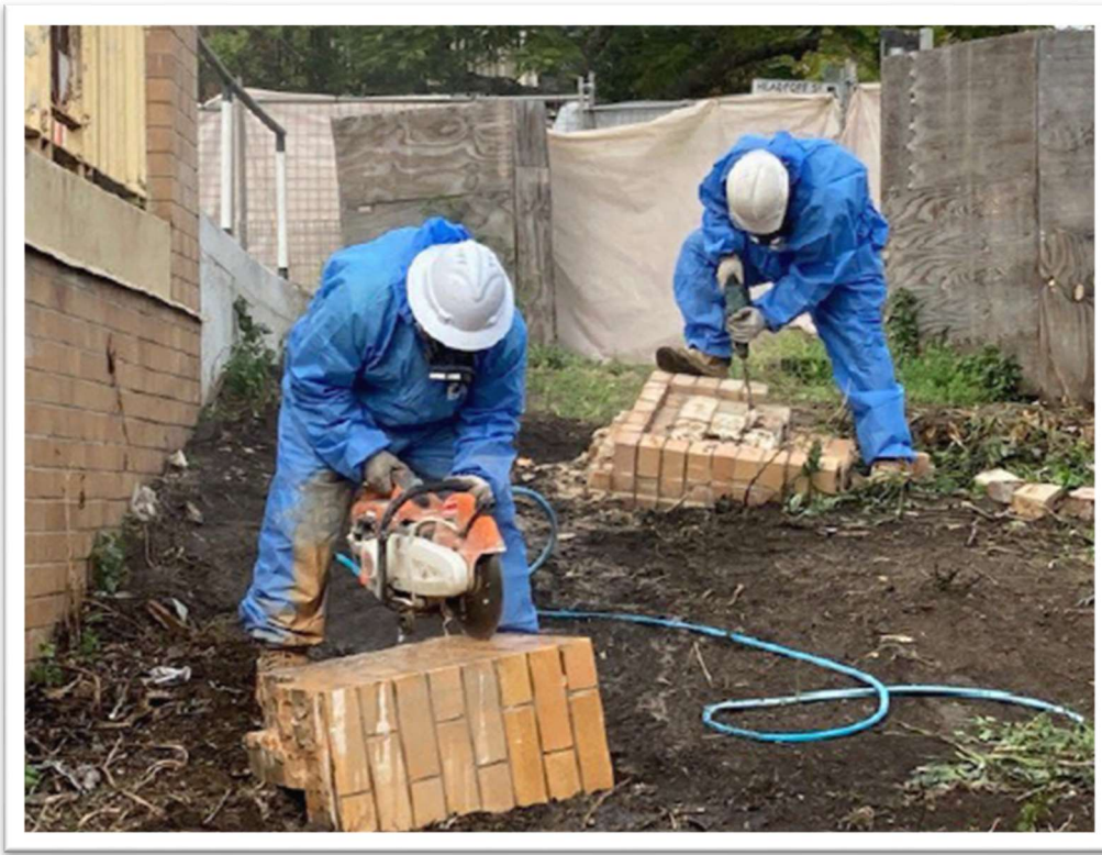
Figure 13. “WET” SAW & MANUAL SEPARATION METHODOLOGY OF THE BRICK COLUMN SECTIONS.
