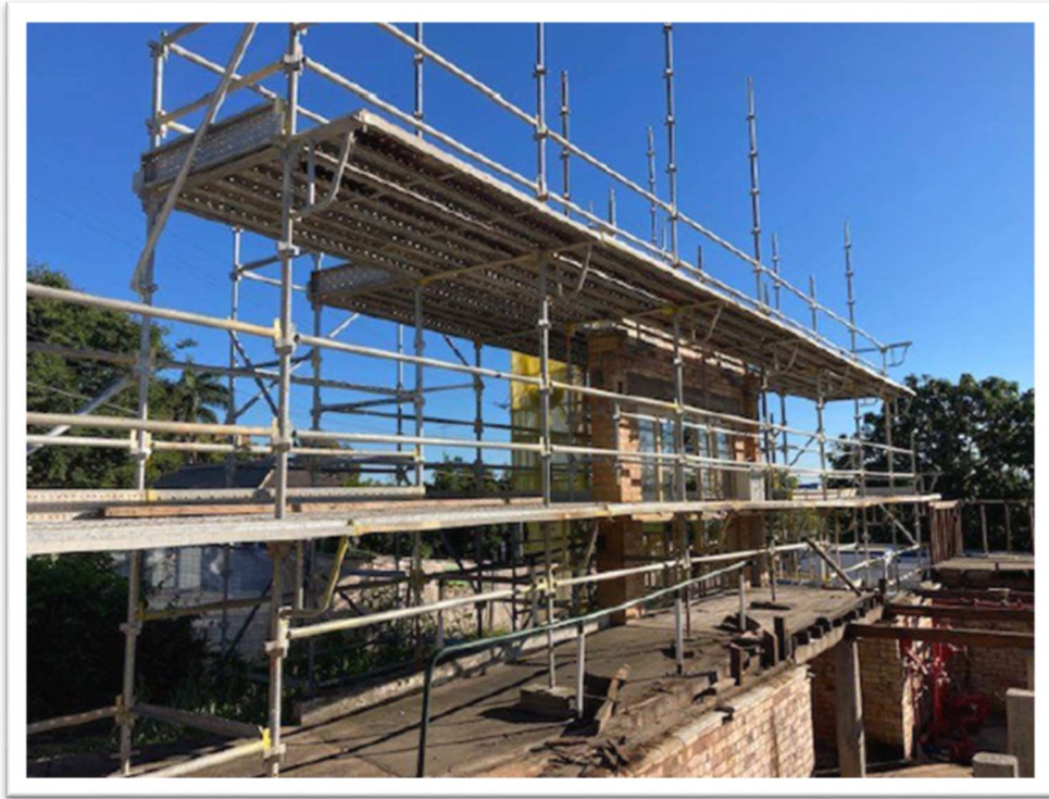
Figure 6. PORTICO SCAFFOLDED AND READY FOR DECONSTRUCTION.
