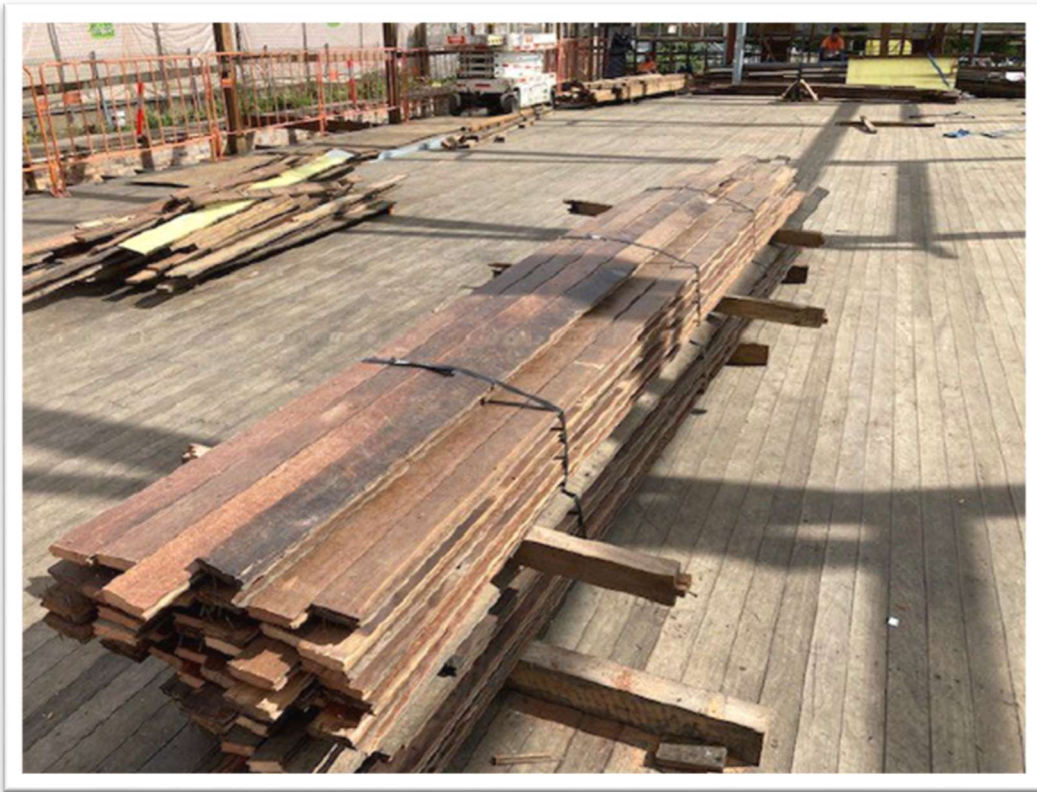
Figure 31. SALVAGED T&G FLOORING, STACKED AND WRAPPED READY FOR DELIVERY TO BCC OFF-SITE STORAGE.
