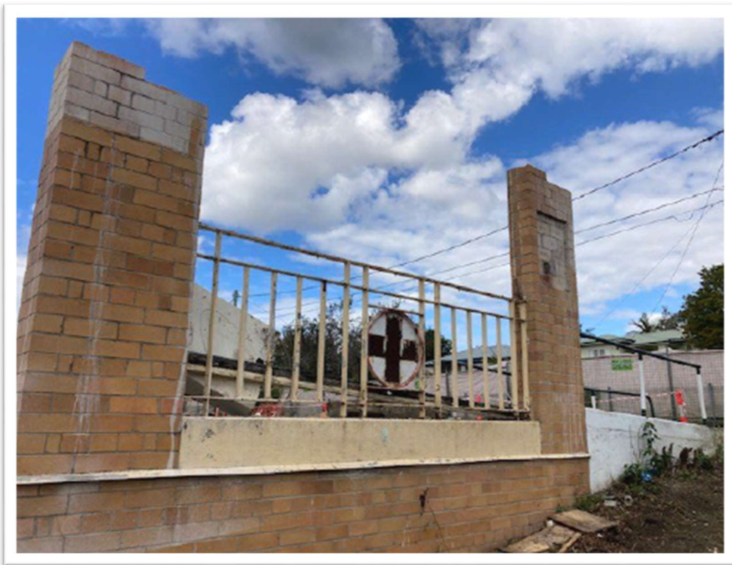
Figure 11. REMAINING PORTICO FOLLOWING THE SALVAGE OF THE HEAD STOCK BRICKWORK AND THE REMOVAL OF THE ACCESS SCAFFOLDING.
