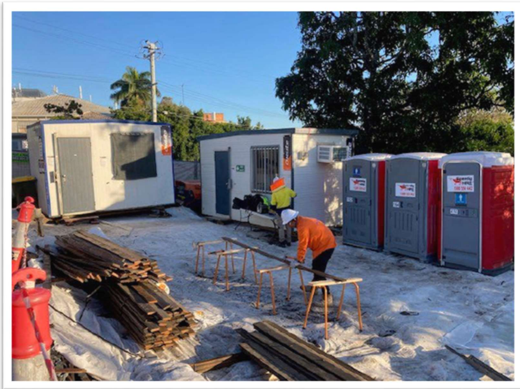
Figure 33. DE-NAILING OF SALVAGED FLOORING.
