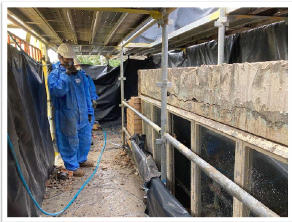
Figure 7. BRICK PORTICO RECOVERY WORKERS IN RPE (P2/P3 HALF FACE) AND TYPE 5/6 DISPOSABLE COVERALLS DUE TO SILICA DUST RISK.
